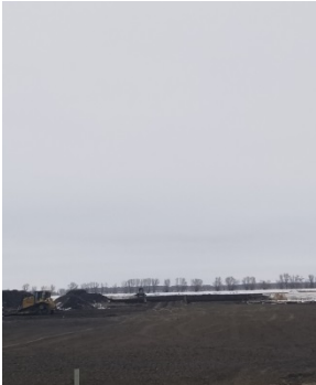
SSKP 1047 North of HWY 3, soil replacement Photo taken North
